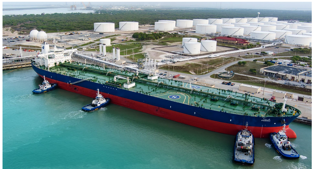
Enbridge Ingleside Energy Center (EIEC) near Corpus Christi, Texas
